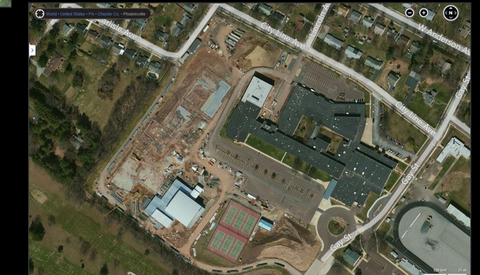
Site Under Construction
